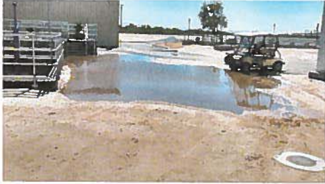
Figure 1 West Side of Flocculators
