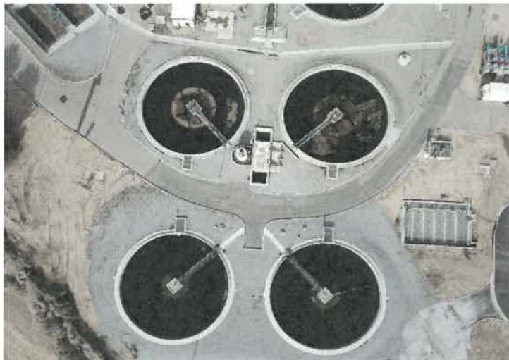
Regional Secondary Clarifiers
