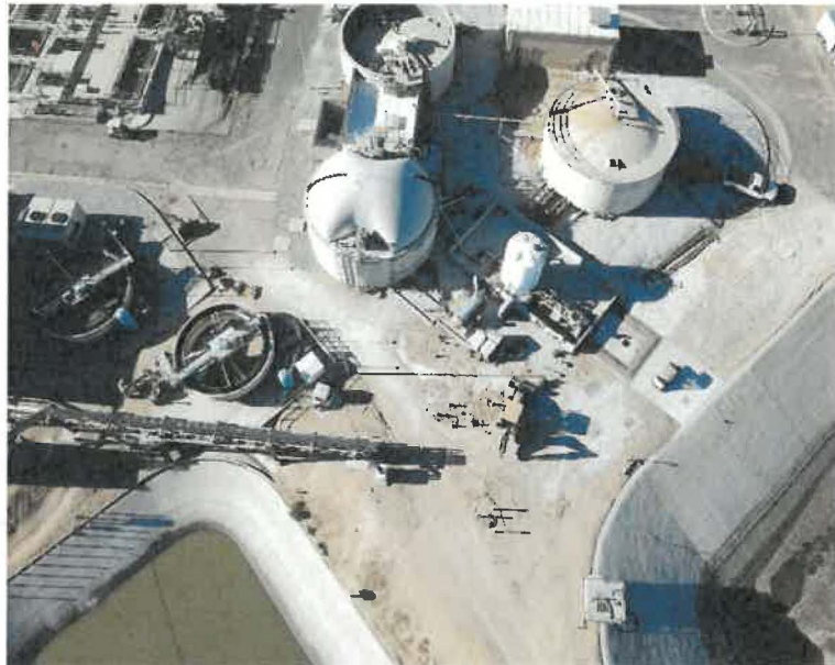
Regional Plant Digesters
