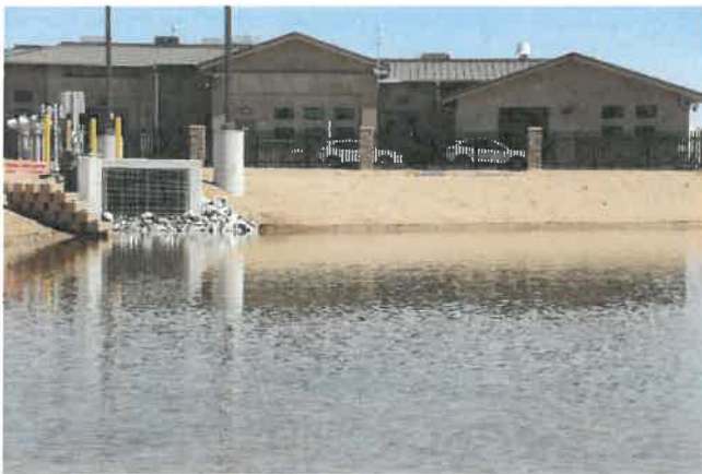
Hesperia Wastewater Reclamation Plant
