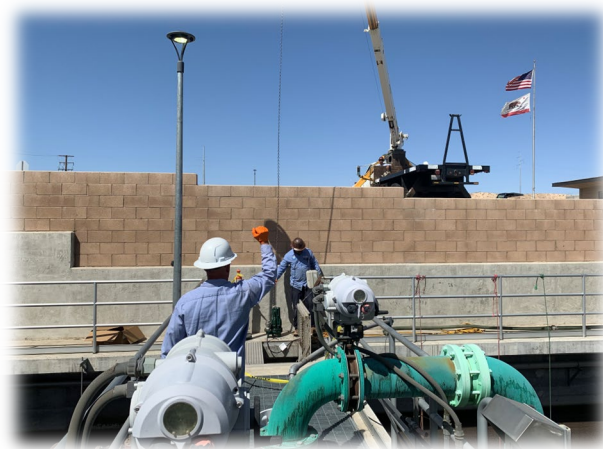
Hesperia Sub-Regional Plant
